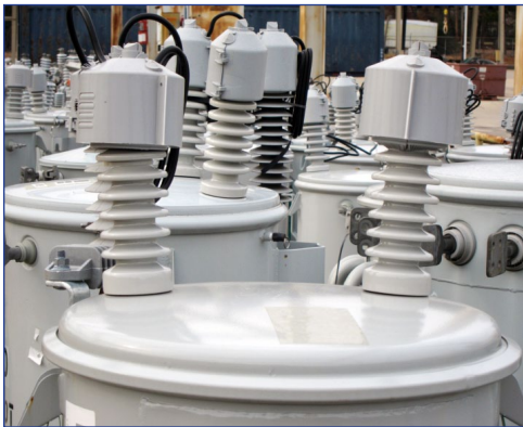
Large yards and multiple-location operations benefit from automated, real-time data collection and distribution
